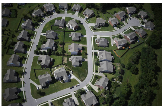
An aerial view of residential neighborhoods containing rental properties in Spring Hill, Tenn. Financial firms are turning to broker price opinions, or BPOs, as a quicker and cheaper way to appraise home values. PHOTO: LUKE SHARRETT FOR THE WALL STREET JOURNAL
